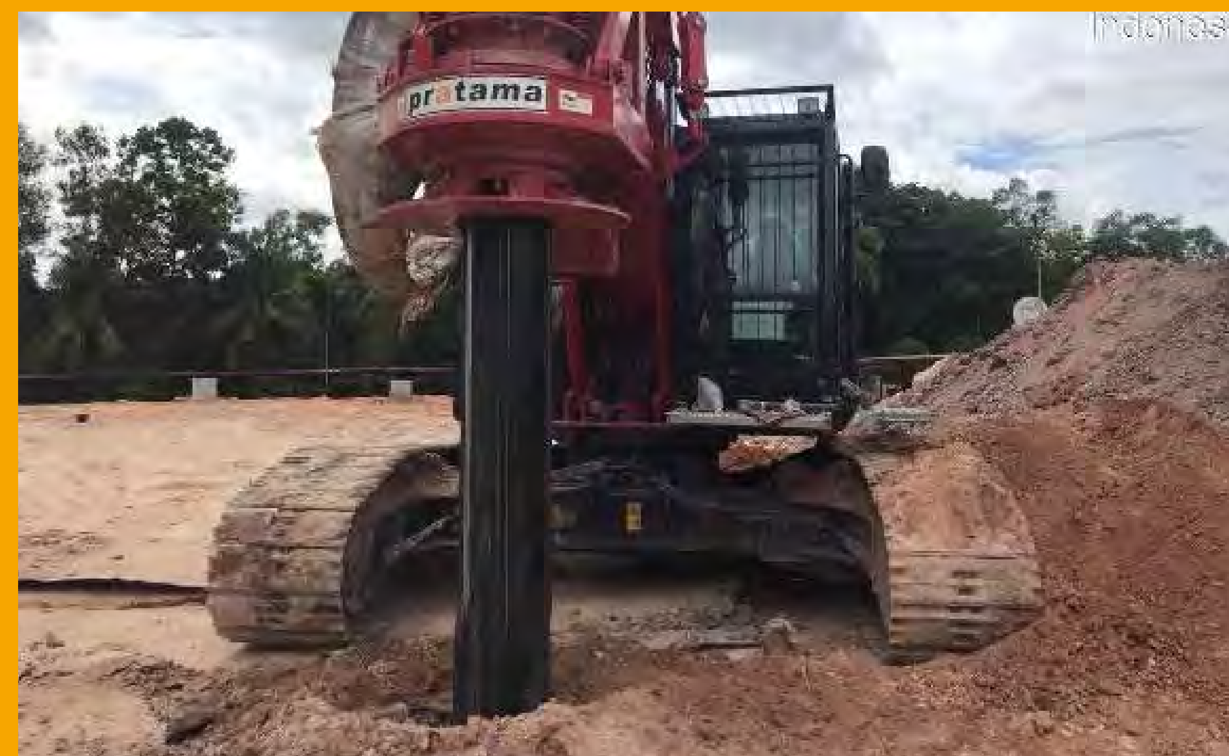
Boredpile Construction of UIB Rectorate Building
