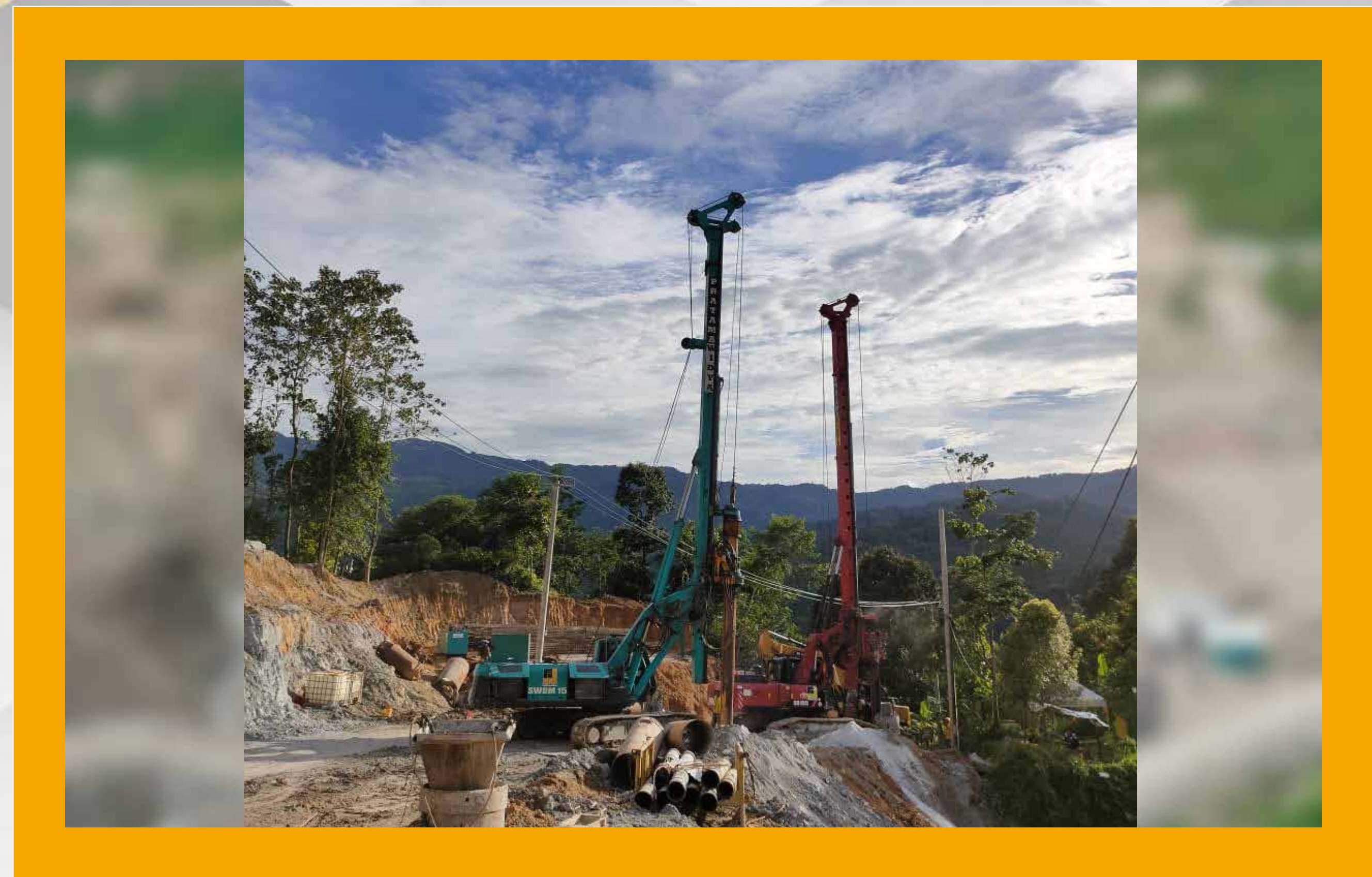
Bored Pile of Cipanas Road and Bridge Rehabilitation Project - Warung Banten
