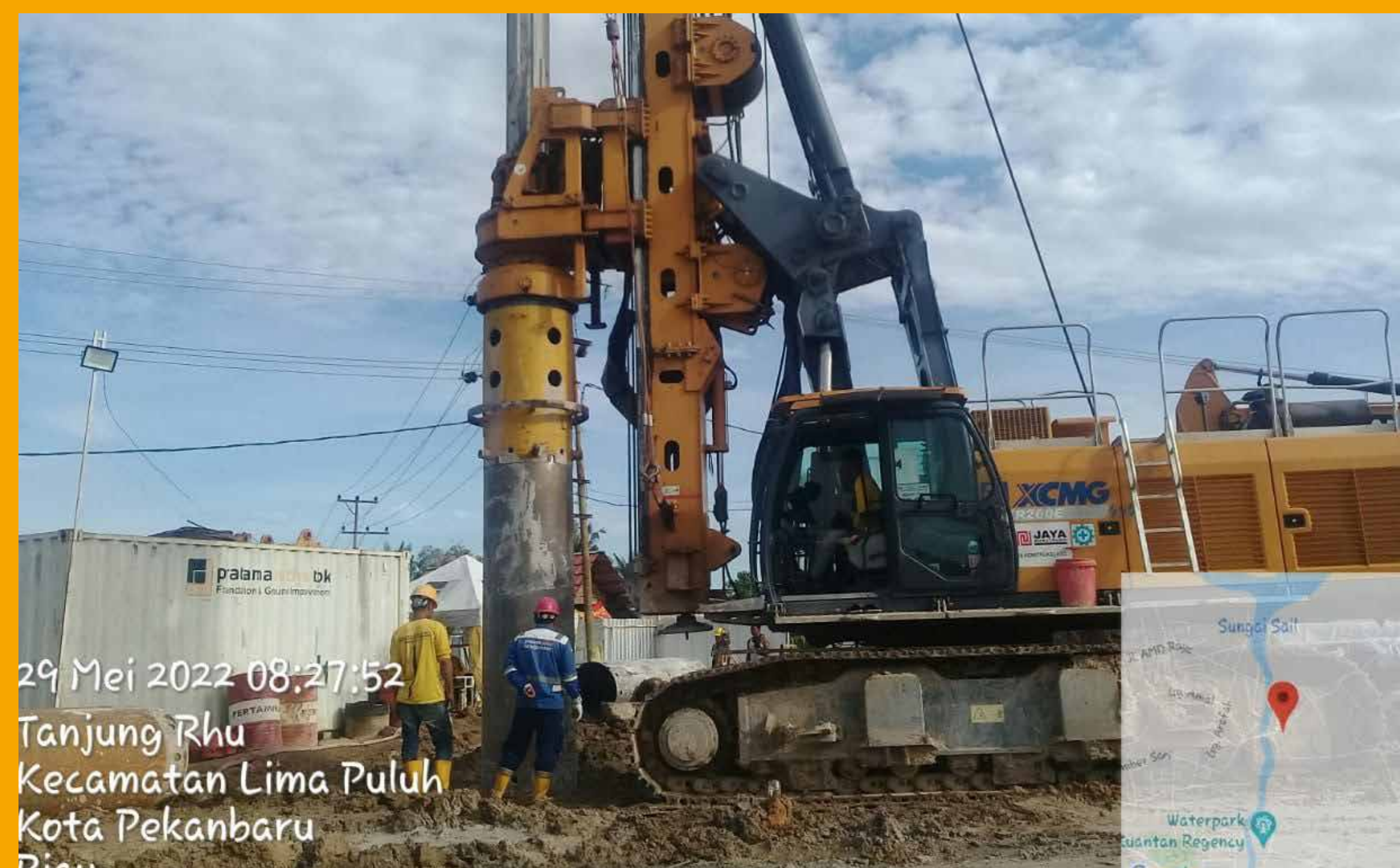
Secant Pile Project Construction of the North Zone Waste-water Piping of Pekanbaru City
