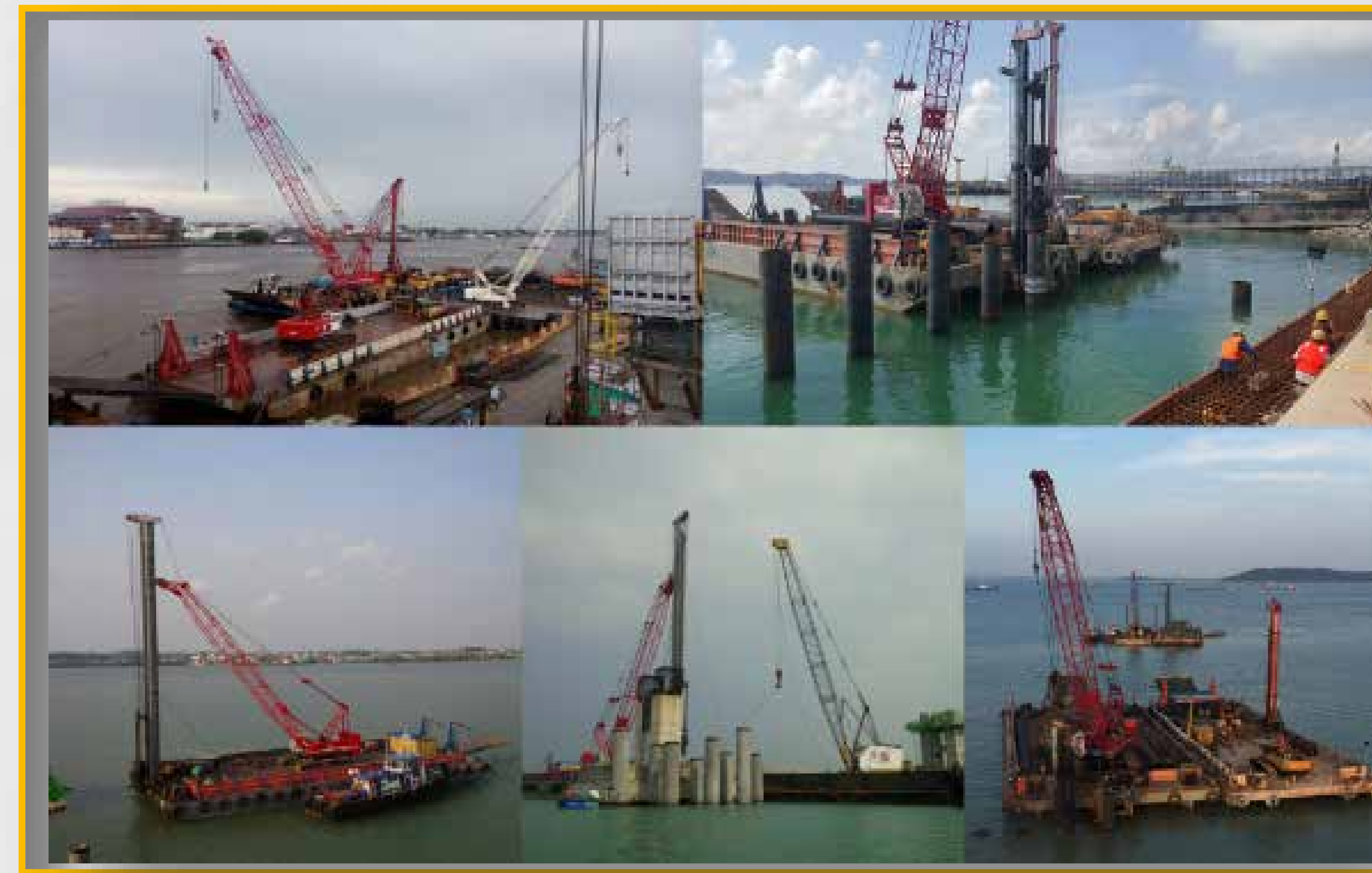
Foundation & Retaining Wall
