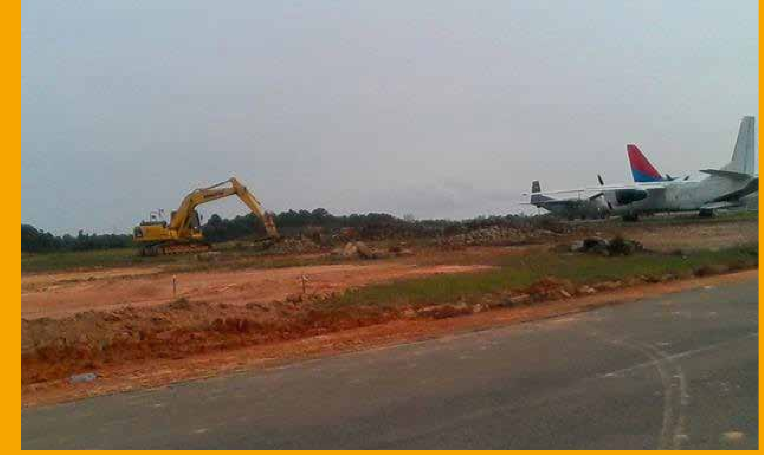
Airport Project Piling
