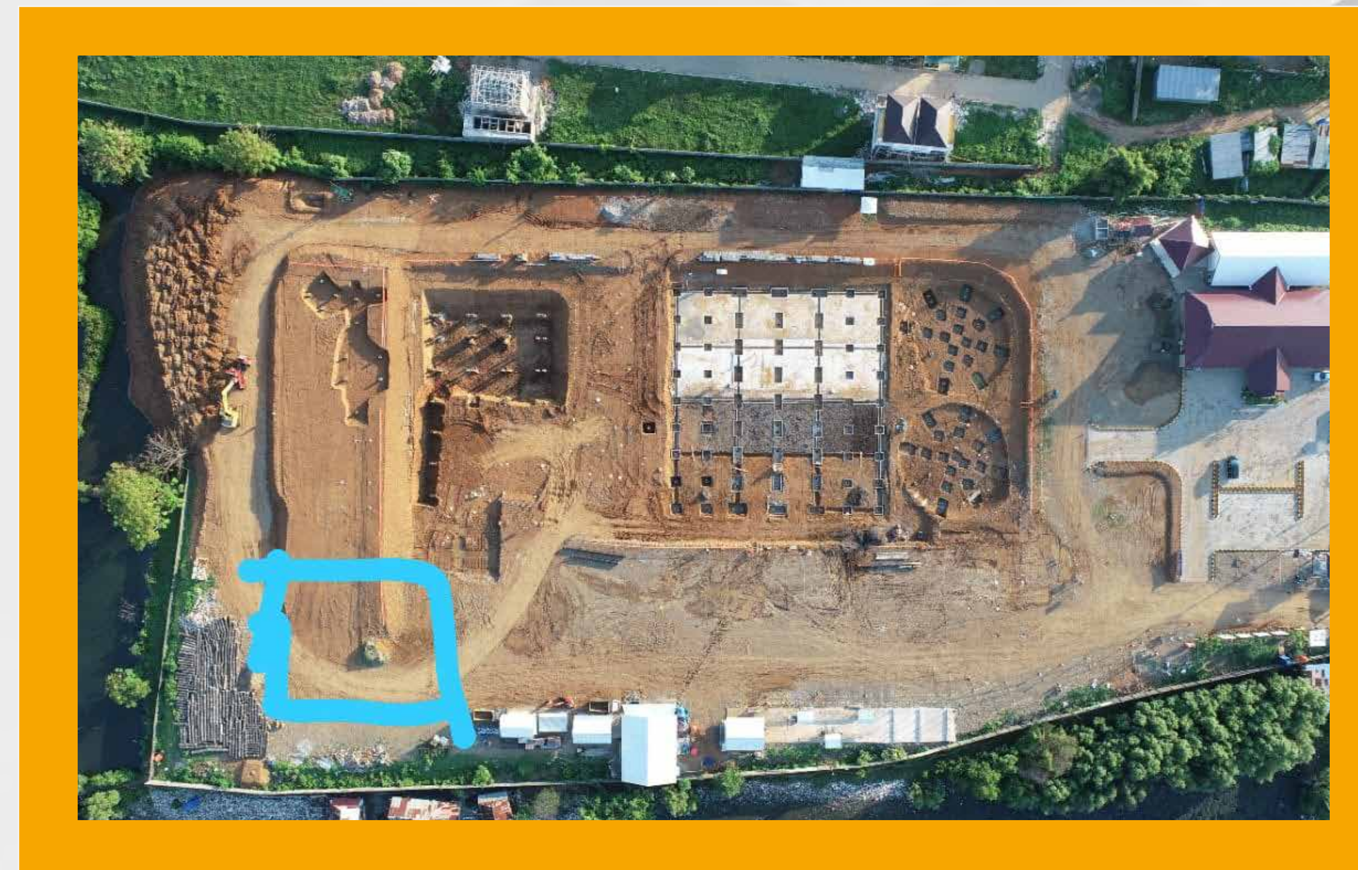
Diaphragm Wall - WWTP B1 Makassar
