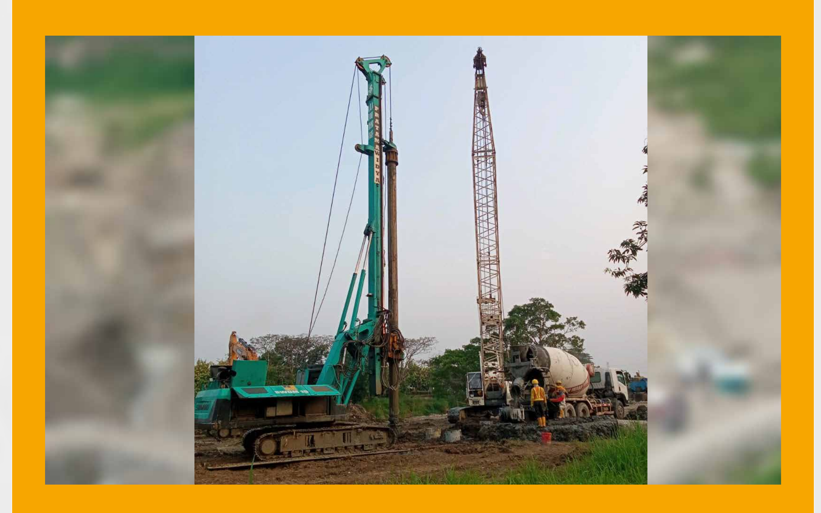
Bored Pile Bekasi River Flood Control Project Package 1
